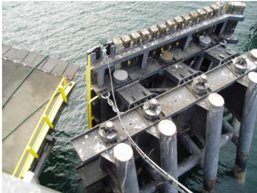
Wing Wall Ground Anchors Figure 26
