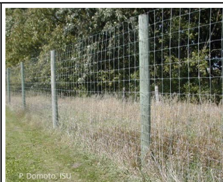
Figure 104. Permanent woven-wire deer barrier.
